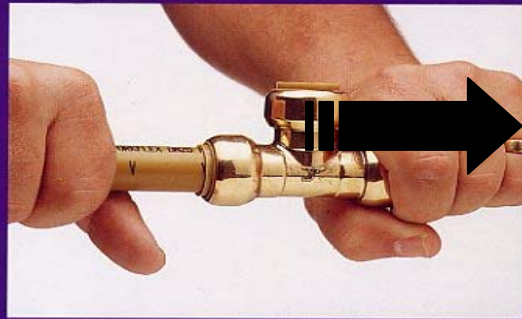
Push the tube firmly with a twisting action until it reaches the next Safe Seal Indicator Mark.
