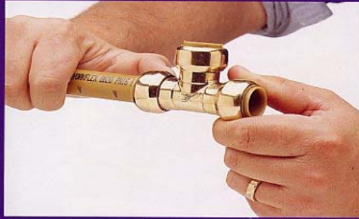
Insert the tube through the release collar to rest against the grab ring.
